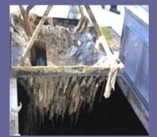
This is a picture of a sewer catch screen. It catches bigger objects as wastewater passes through it on its way to the treatment plant. The stuff you see here is a collection of paper towels, wipes and other non-disposable products that could not pass through the screen. CFPUA has 140 pump stations which utility workers clean out every.
