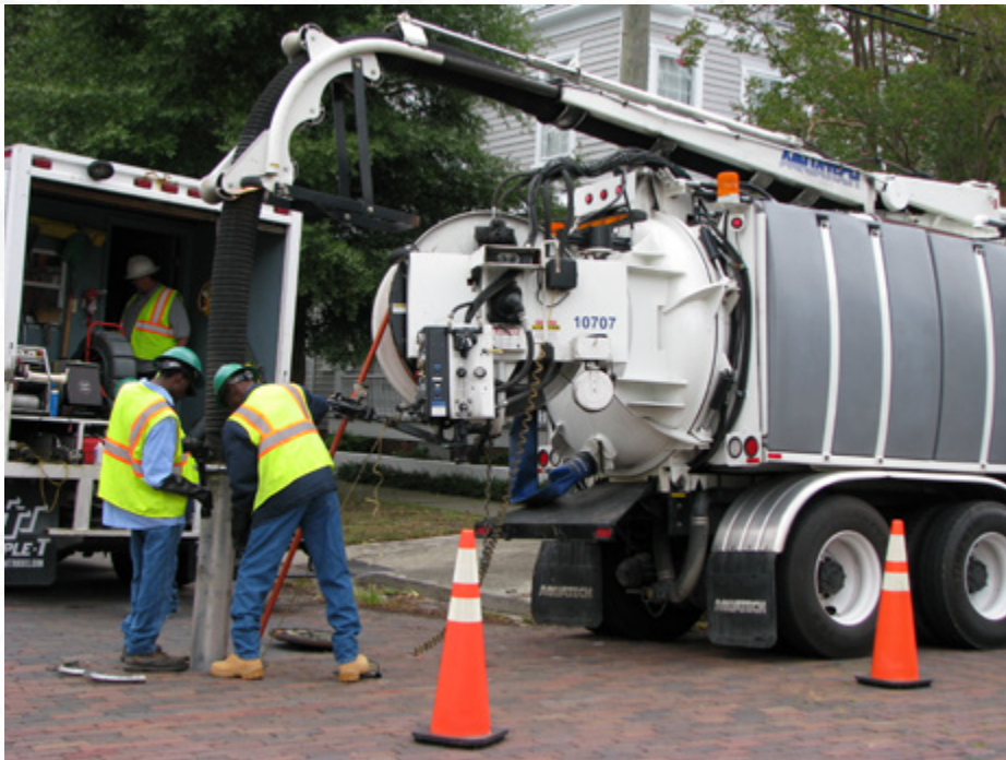
Sewer System Maintenance
