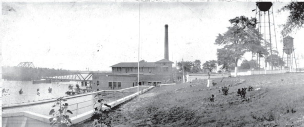
Clarendon Water Works, 1908
