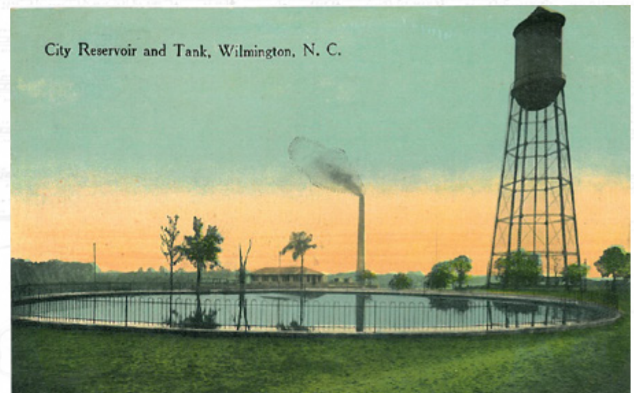
Clarendon water works, early 1900s
