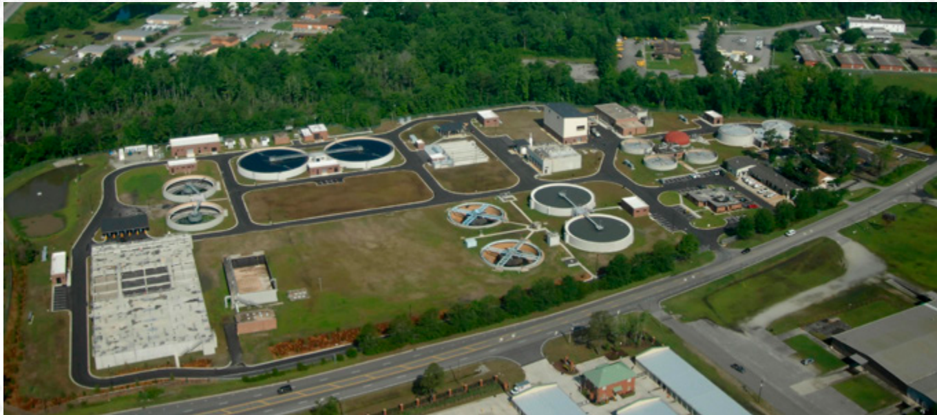
James A. Loughlin (Northside) Wastewater Treatment Plant
