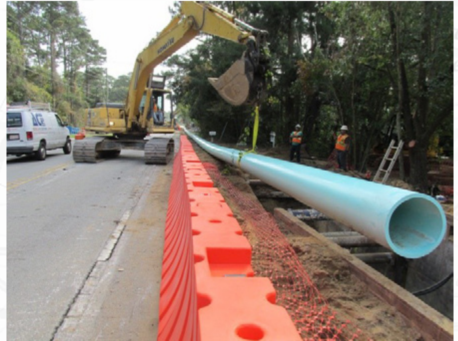
Northeast Interceptor Rehabilitation
