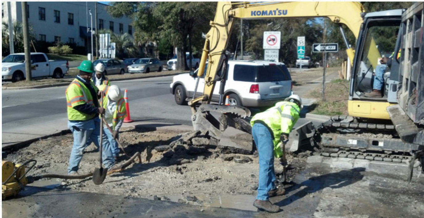
Water Main Repair Work
