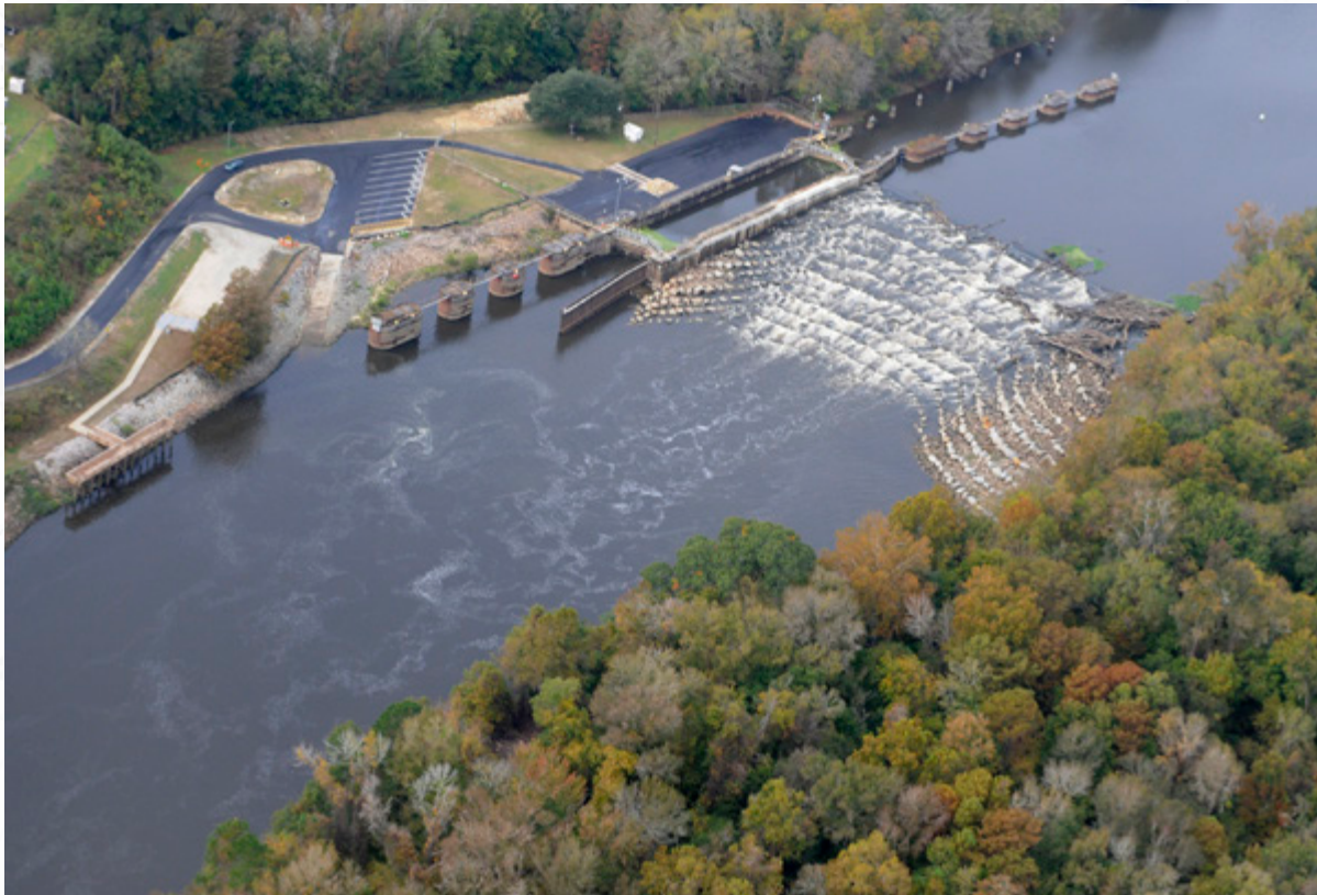
Lock and Dam #1
