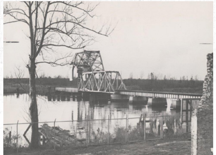
Smith Creek Bridge
