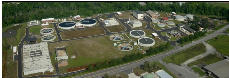
Northside Wastewater Treatment Plant
