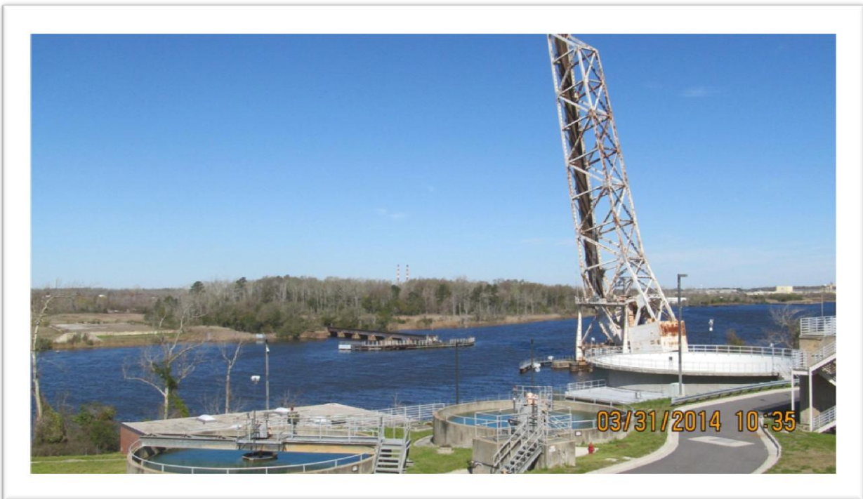
Photographer: Sam Yarboro, Sweeney Water Treatment Plant
