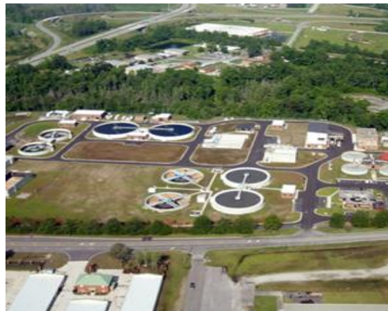
Northside Wastewater Treatment Plant
